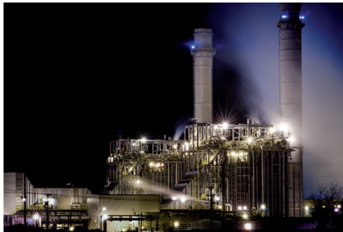
Gas naturaleko zentral elektriko bat, Oregonen. ARG. SCOTT BUTNER PHOTOGRAPHY/LLC.
